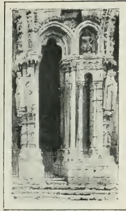
FIG. 127.—DETAIL OF THE NORTH PORCH OF THE CATHEDRAL OF CHARTRES.
