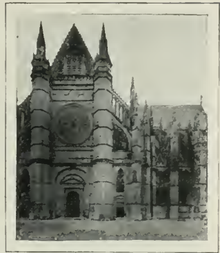
FIG. 3-1.—ORLEANS CATHEDRAL, SOUTH PORCH.
