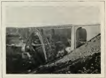
FIG. 812.—THE VIADUCT AT GARABIT.
