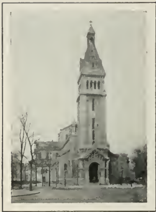
FIG. 705. VAUDREMLER. CHURCH OF SAINT-PIERRE AT MONTROUGE.
