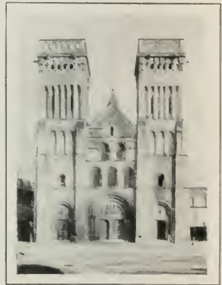
FIG. 38. — FACADE OF LA TRINITÉ (ABBAYE AUX DAMES), AT CAEN.
